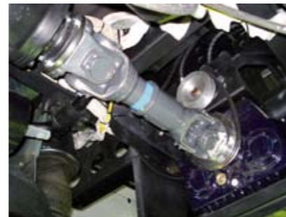
Installing traction engines and mechanical couplings onto the traction axle.
